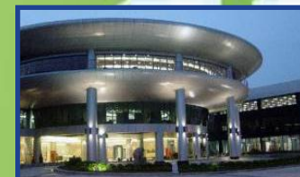
China Technology Center Shanghai, China
